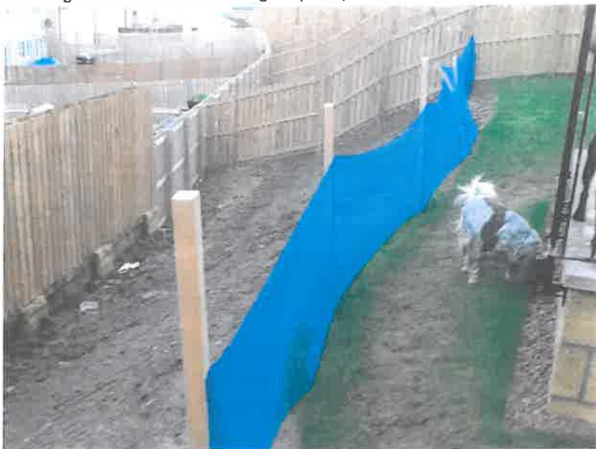
View of garden before deck showing the patio platform to RHS;-
